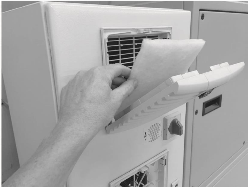
Fig. 93: Filter replacement in control cabinet
