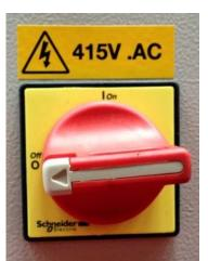
Also, on the door of the control panel is an Electrical Isolation Switch 4. The switch must be turned to the off position, cutting power to the panel in order to open the door. The handle can also accept a padlock or similar, in order to lock out the panel and prevent it from being powered up.3.2 Control Pendant Operation
